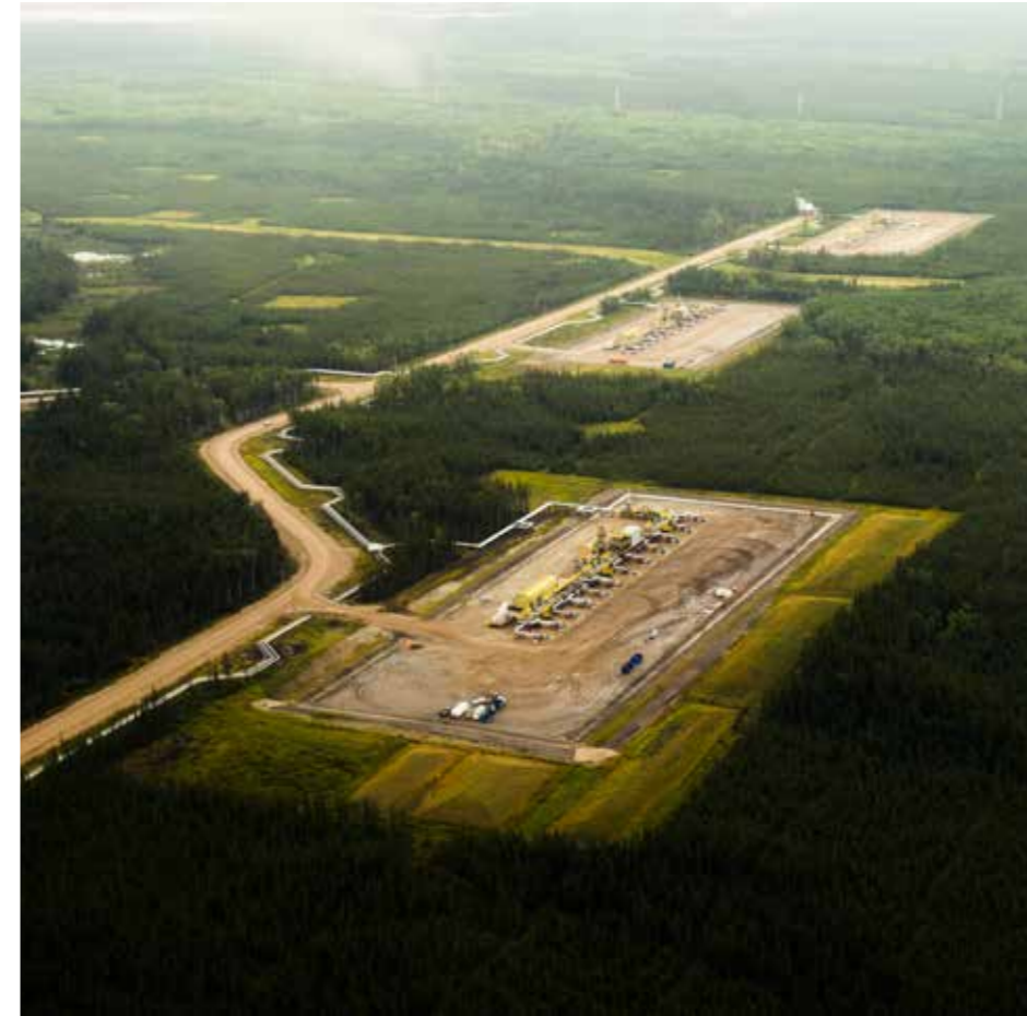
Canada's Bitumen Landscapes - In-Situ Extraction Well-Pads These images show well-pads where bitumen is being extracted from deep underground. It is also possible to see the many pipelines taking steam to the site, and diluted bitumen away from the site for processing. (All images Christina Milos 2015)
