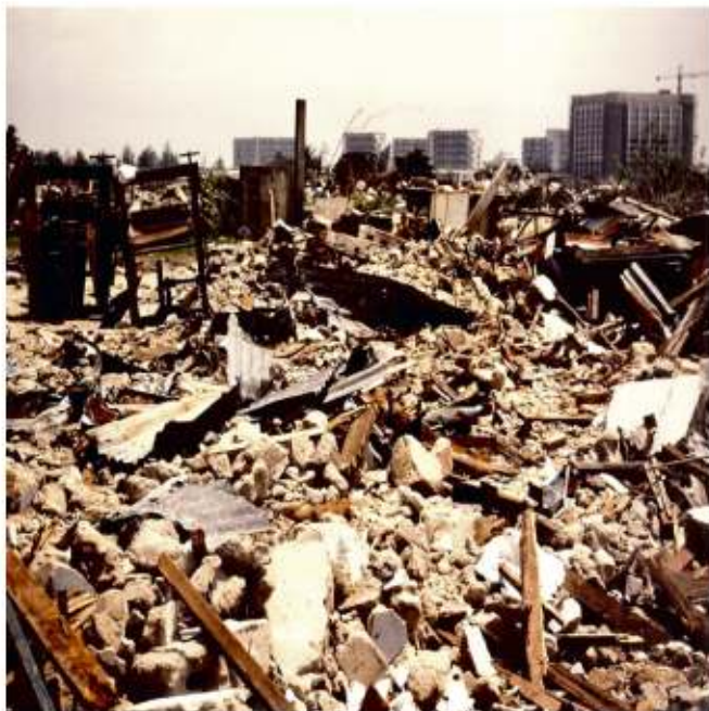
Demolition of Maroko 1992. Photo: Renate Albertsen-Martton
