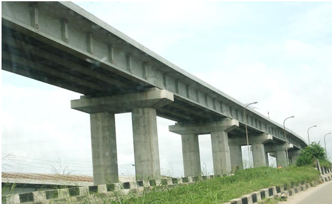
Fig. 4 The Lagos Light Rail facility under construction
