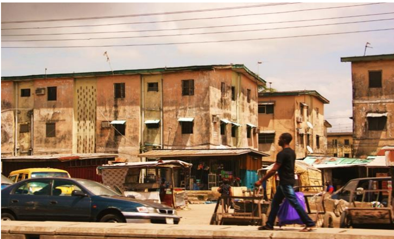
Fig. 9 Jakande Housing Estate
