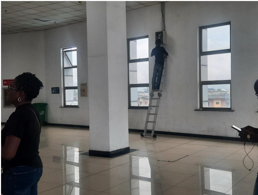
Figure 9. Ongoing maintenance at Mile 2 station. Photo credit: Israel Faleye.
