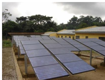
5.5 kWp Solar PV plant at Laje in Ondo State (picture: Prof. Sambo, Energy Commission of Nigeria)
